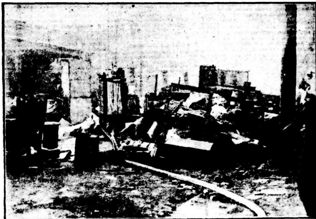
When the fire broke out in Messrs. Milburn & Jeffery's joinery works in North-street, Adelaide, on Saturday afternoon, the neighboring houses were threatened with destruction and the occupants hurriedly removed their furniture and personal belongings. The photograph shows some of this impedimenta in North-street. F. M. Gray, photo.
