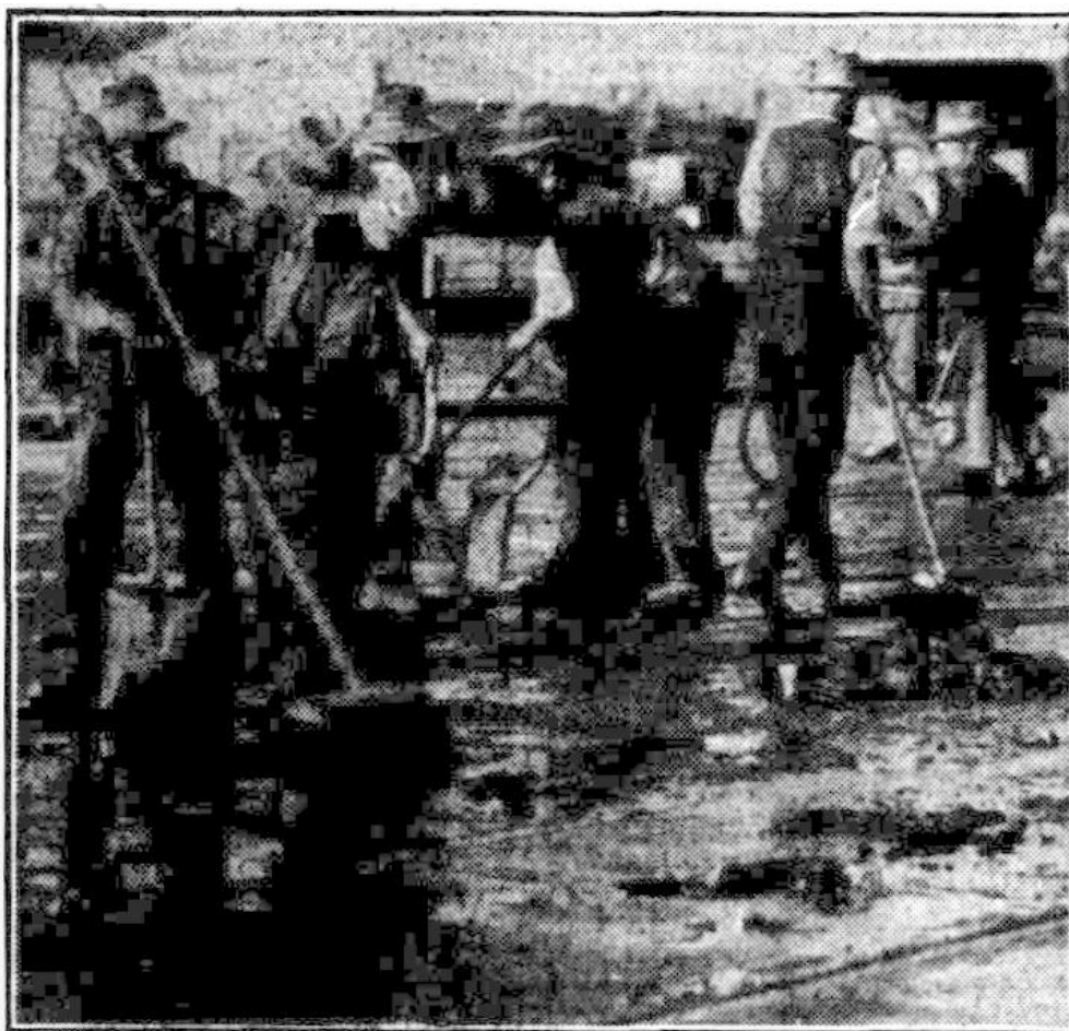
ROAD ON FIRE.—Liquid bitumen accidentally flowed from a bitumen wagon at Hindmarsh Square on Monday afternoon and caught fire. The road blazed fiercely until the Fire Brigade put out the fire.
